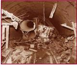
were working in the tunnel at the time of the blast were killed. The tunnel, located under the grounds of Fort Gratiot County Park, was being constructed to provide drinking water for the City of Detroit and Southeastern Michigan.
